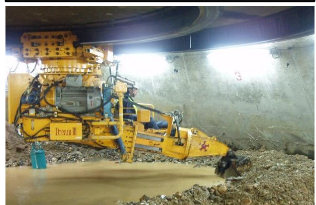
④掘削・沈設
